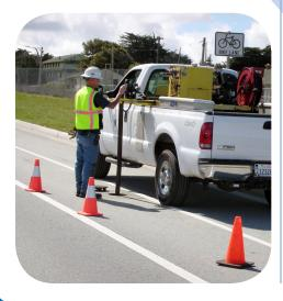
Water valves require exercising to comply with California Department of Health regulations and to ensure these vital assets operate when needed. During emergencies, it can be necessary to turn off the water to prevent damage and to facilitate repairs. The water valves are the critical component to accomplish this quickly and efficiently.
